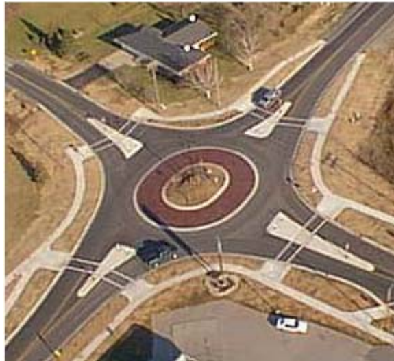
Figure 1.1 Modern Roundabout, Brown County, Wisconsin
